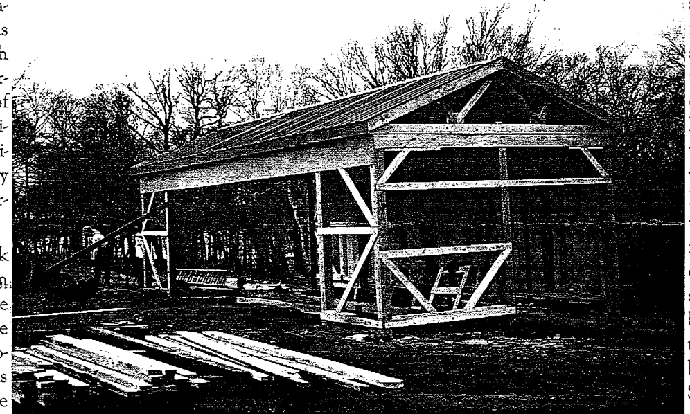
The Woodmizer Shed during construction. (11/00)
